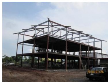
Structure framing finished Aug, 2010
