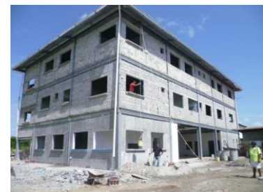
Exterior completion Feb. 2011
